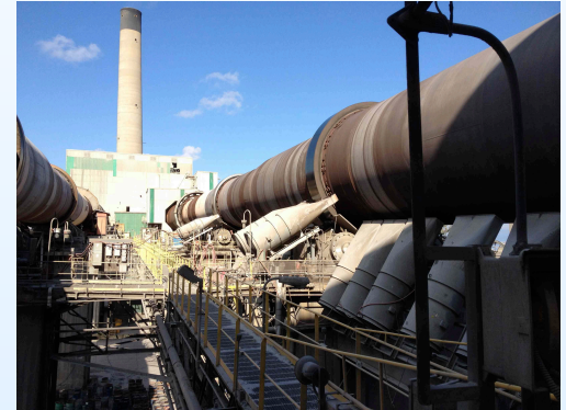
Portland Cement Manufacturing Ravena, NY
